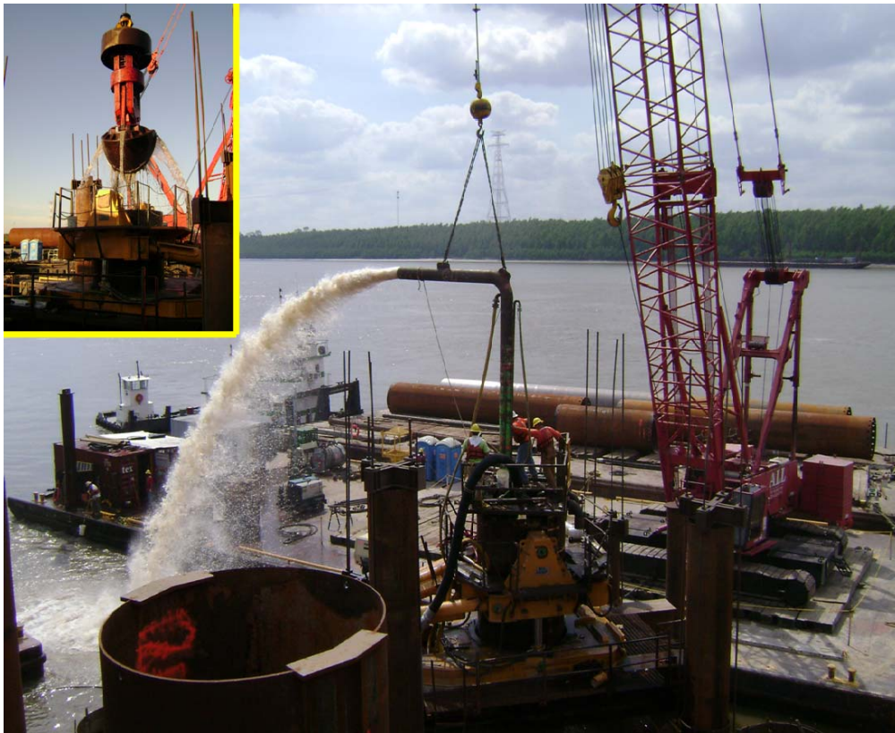
Figure 2. Shaft Excavation Using Oscillator, Grabs, and Air-lift.
