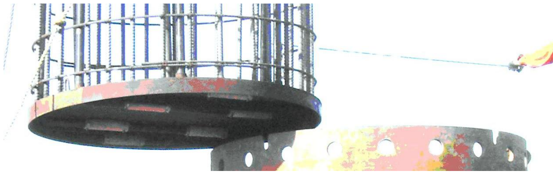
Figure 3. Sleeve-Port with Top Plate Grouting Mechanism.
